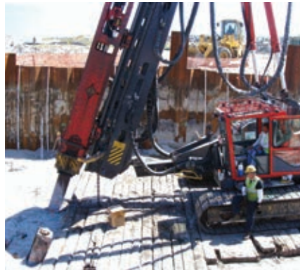
CCO Pile Driver operator certification is slated for early 2016 launch
